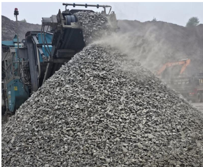
Sub-Base and Structural Fill
