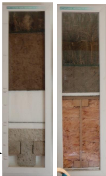
Green Roofs with thick insulation
